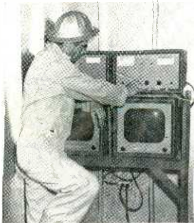
Twin viewing screens located in control house aboard tower barge
