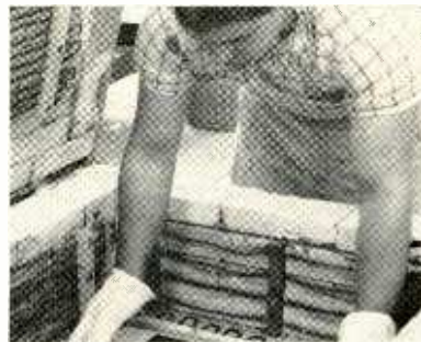
Group of etched-apart parts are given final heat treatment
